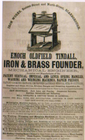
Above Washing machines for Scarborough's landladies.
