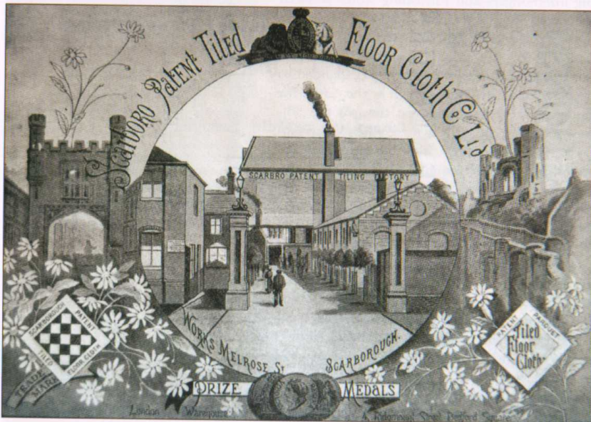
Below The new Scarborough linoleum made for boarding house floors.
